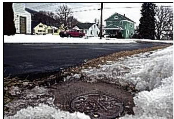
A monitoring well, bottom, outside a house on Map Street in Vestal. An MTBE spill in this neighborhood is one of 29 in Broome County.
