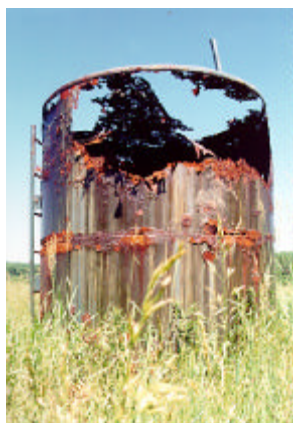
A brine tank in Chautauqua County in need of repair.
