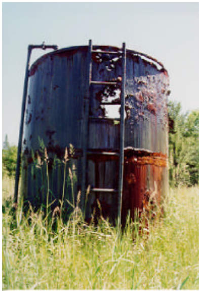
A brine holding tank in the Town of Gerry, Chautauqua County.
