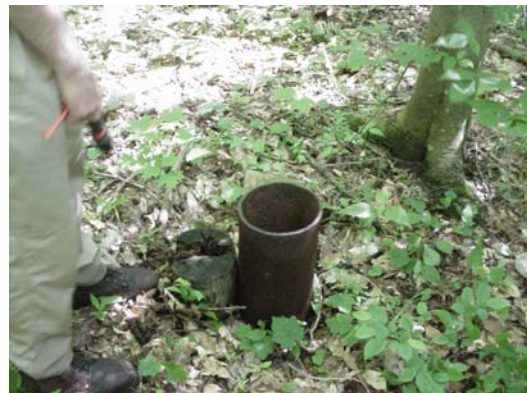
Photo 4. This leaking gas well on State land is a safety problem. Abandoned wells can also cause oil leaks, kill vegetation and contaminate ground and surface waters with oil, gas or brine.
