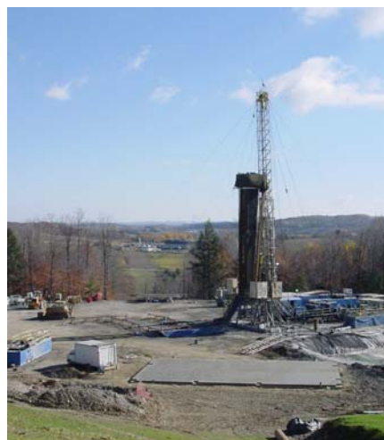
Photo 8. Drilling of a new storage well at the Stagecoach Field.
