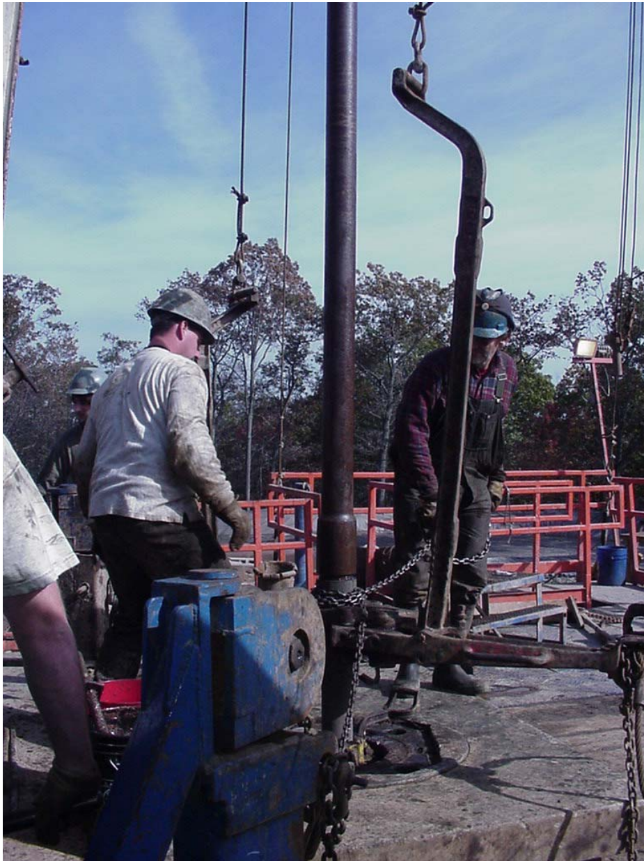
The rig crew is making a drill pipe connection so they can continue drilling this well on a State lease in Schuyler County.
