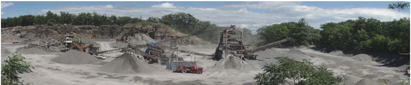
Processing equipment similar to this screen and wash plant allows mine operators to wash, sort and produce aggregate of varying sizes to meet the required specifications for a job.
