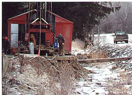
The mostly wooden structure is an older style of drilling rig known as a cable tool rig. It is being used to plug a well in a DOT right-of-way next to a stream.
