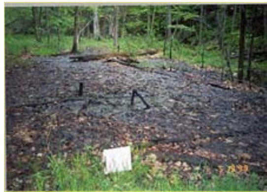
Moore Lease abandoned well near creek leaking crude oil to water.
