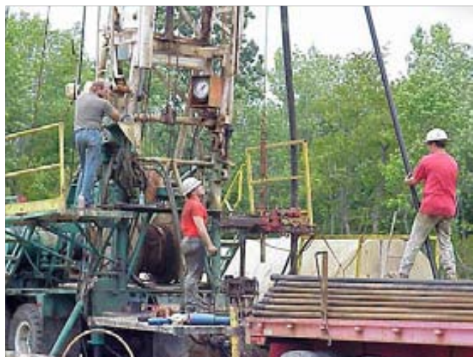
Rig crew plugging and abandoning a well.
