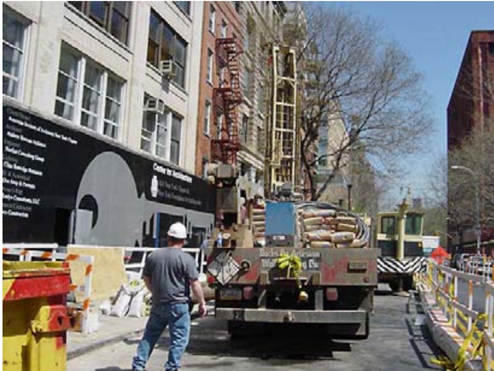
Drilling rig and cement truck on the sidewalk in front of the American Institute of Architects in downtown Manhattan, New York City. The workers are preparing to cement the casing in a geothermal well.
