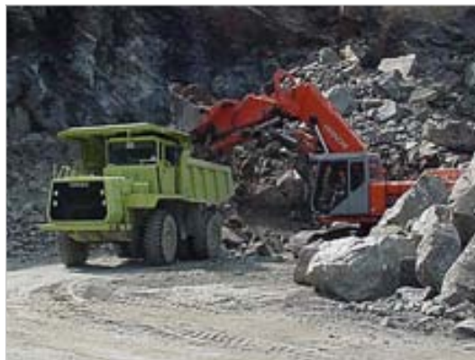
Hydraulic shovel loading dumptruck with rubbleized stone after a blast.
