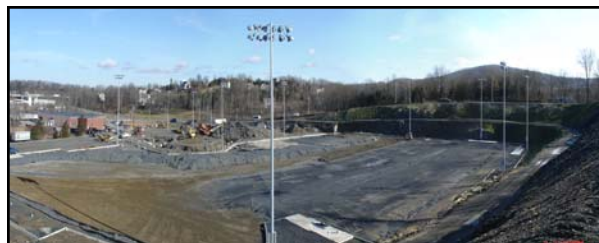
Frozen Ropes site during a December 2009 inspection.
