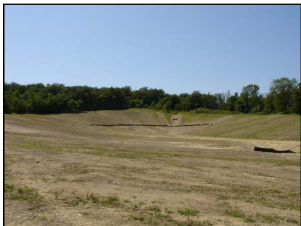
Graded portion of the E. Tetz & Sons-Echo Lake Mine (Town of Goshen, Orange County) during concurrent reclamation operations.
